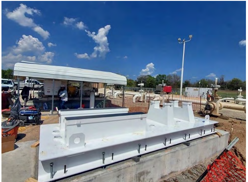
Foundation completed and ready for epoxy grout in 24 hrs. This shortened time gap reduces the exposure window where debris, laitance, or moisture could compromise the bond.
