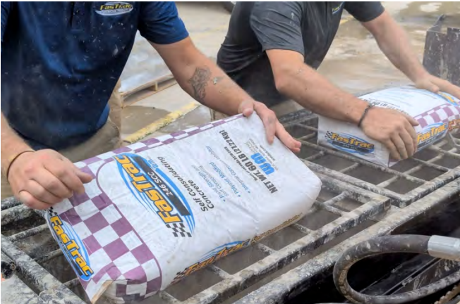
FasTrac 246 SCC was mixed on-site using the FasTrac 750 Skid Steer Mixer. The mixer includes a pair of bag-breakers on the grate for convenience.
