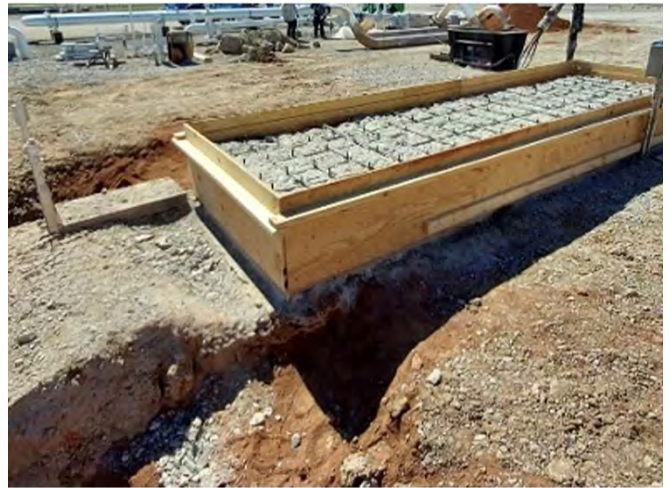
Contractor chipped down to top mat of rebar to ensure proper placement of mechanical pins using CE308 to secure. Form boards placed and prepped for 246 SCC.
