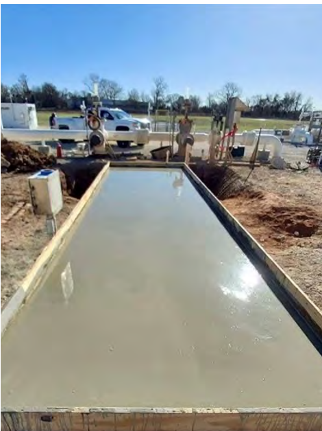
246 SCC placed before new anchor bolts were core drilled and installed with CE308.
