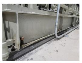
The CE815 Epoxy Grout's excellent side to side flow with limited head pressure allowed for placement in a tight location. The extended working time (>60 minutes) allowed the contractor plenty of time to place the grout and finish the surfaces. The combination of CE815 Epoxy Grout and a professional grouting contractor turned a difficult environment into a routine grouting project.
