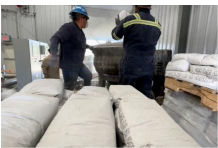
Properly conditioned material and equipment is a key element of a successful grout installation. FasTrac CE815 Epoxy Grout should be conditioned to a temperature between 65-95° F for 24 hours with optimal temperature between 75-85°. All equipment and surfaces should be conditioned to 60-90°.
