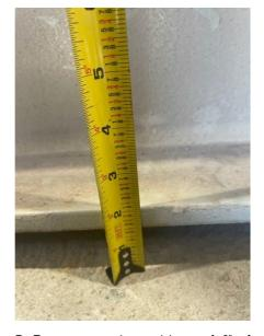
FasTrac recommends a minimum of 2" of clearance between the top of concrete and the bottom of the skid. When 2" of clearance is not possible then proper preparation is essential. S2W Contracting did an excellent job of heating the building, material, and equipment.
