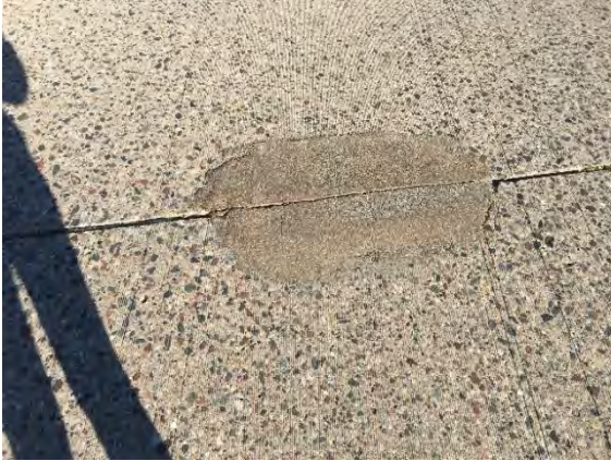
Figure 4.2 Patch Condition Rating = 4 [No Distress]
