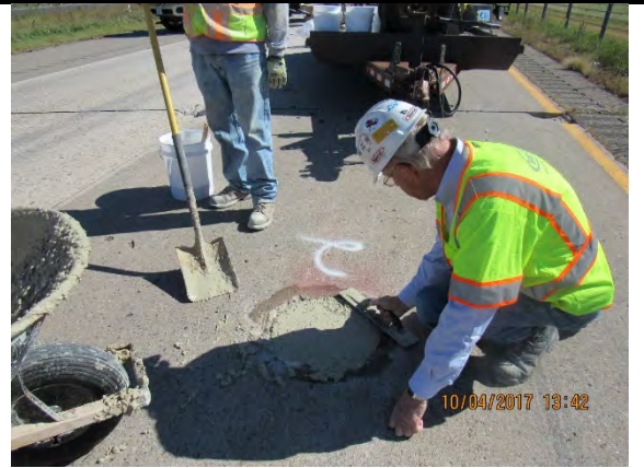
Photograph: 94013 CTS, Rapid set and Helix Fiber Subject: Finishing of products with steel fibers
