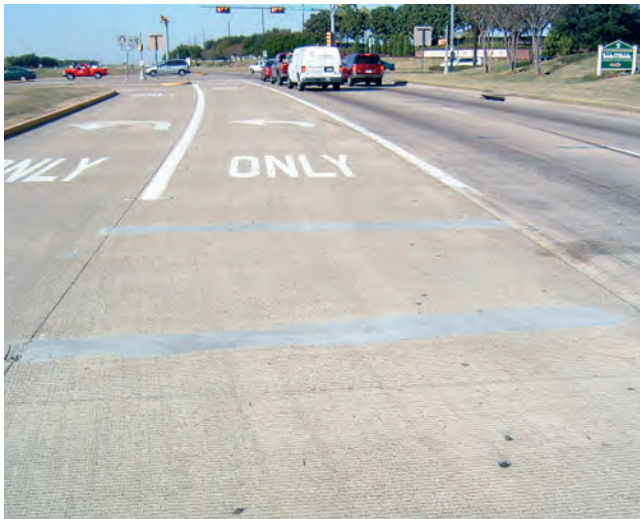
Top and Center images: Highway Spall Repair, Highway 99, Fort Bend County, TX.
