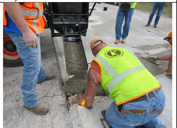
Photograph: 94003 (A) Western Material and Design, FasTrac246 Subject: Concrete placement
