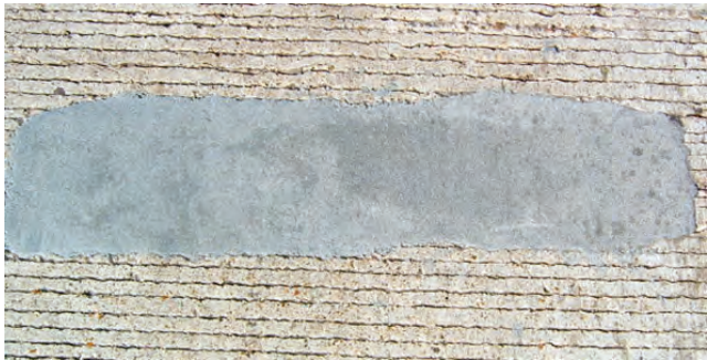
Top and Center images: Highway Spall Repair, Highway 99, Fort Bend County, TX.
